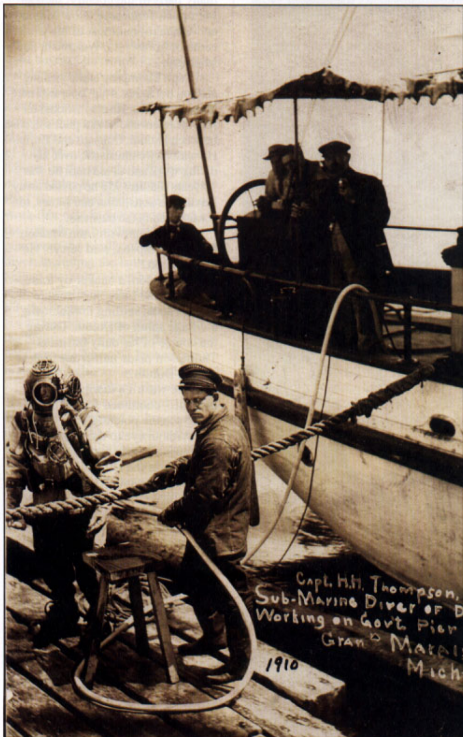
H.H. Thompson at work on the government pier in Grand Marais, Michigan, in 1910.
