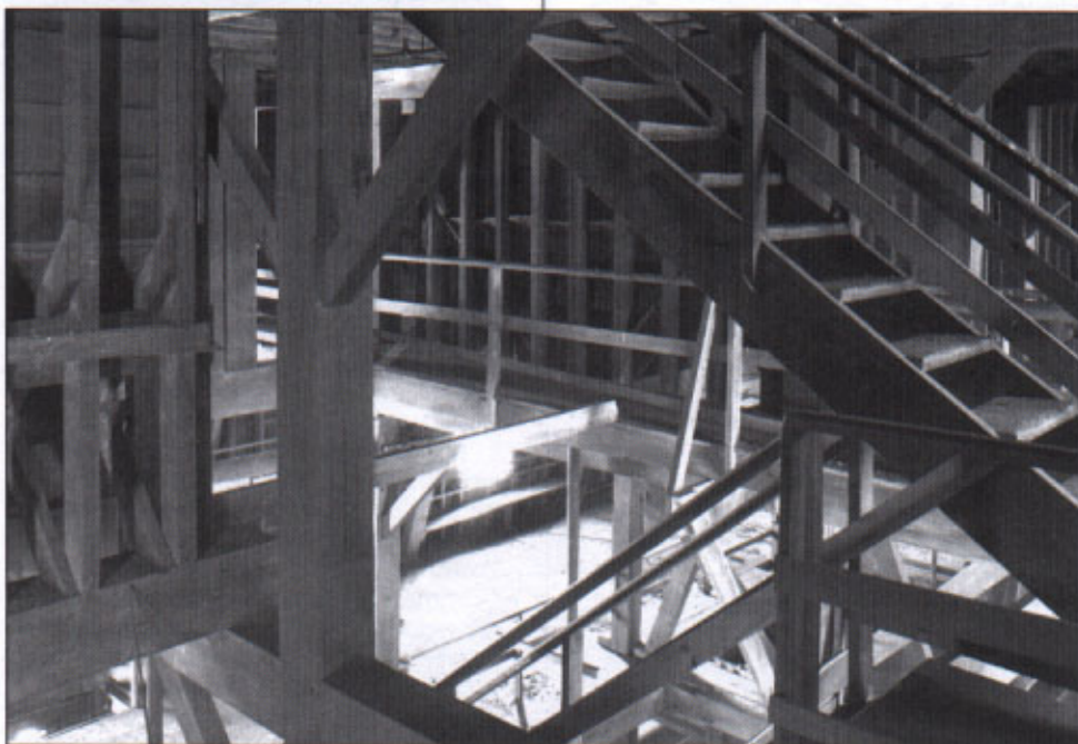
Beams and stairs on "garner floor," showing complexity of wooden-beam construction.
